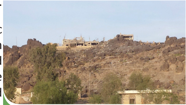
the Seismic Monitoring Center in Hran area
