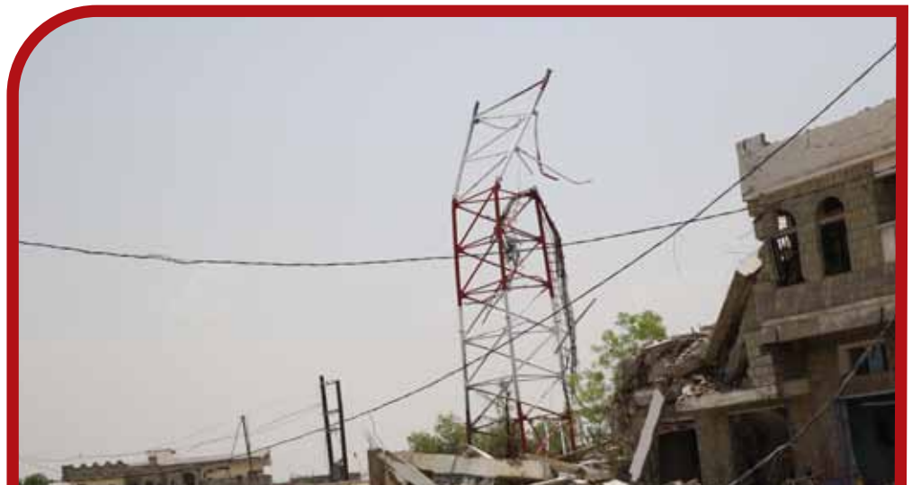
Haradh communication station and network - Hajja province- bombed in 21/4/2015
