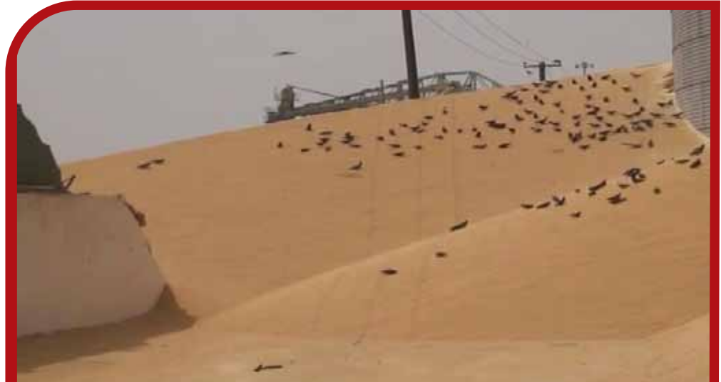
Grain silos –Aden-bombed in 9.4.2015
