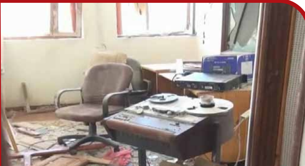
The building of radio in Saada province from inside – 31.5.2015
