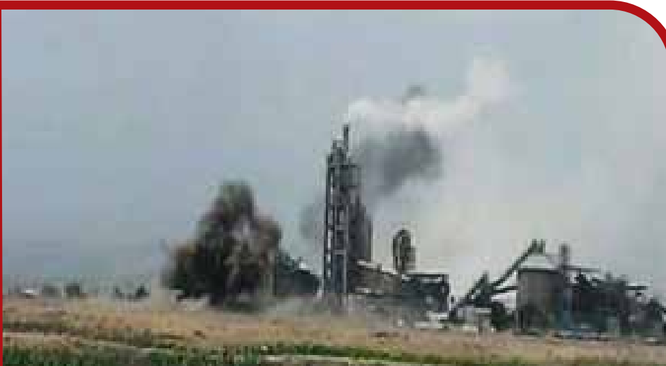
Image for Amran remainder cement factory, bombed in 12/7/2015
