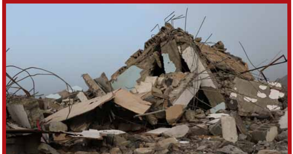
Health center in Mastaba - Hajja - bombed in 27/7/2015
