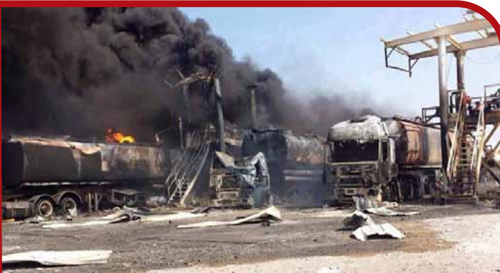
Rass Essa facility - Al-Saleef - Al Hodeida, bombed in 21/1/2016, killed (15) civilians (worker's in the facility) and injured (25) other's.
