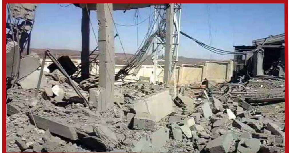
Al-Taiffa communication station and network - Al-Baitha province - bombed in 16/8/2015.
