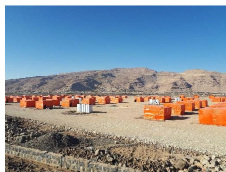
The new IDP hosting site in Kharif district, Amran governorate. Photo: Omar Al Rajawi/ SNC
