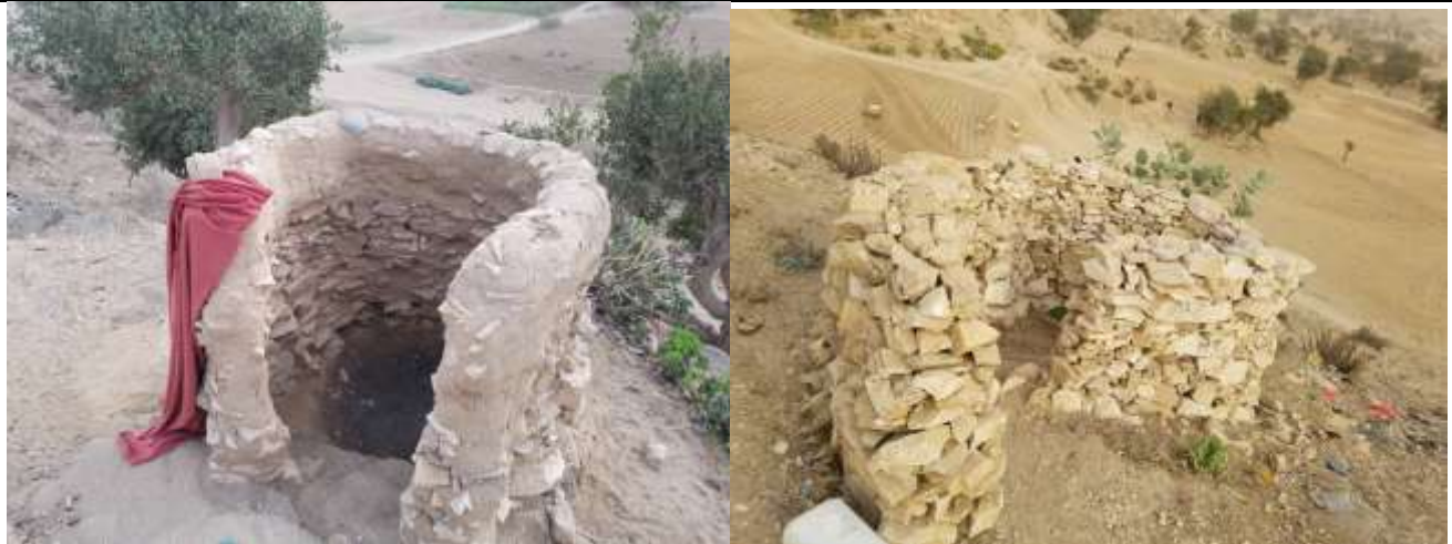
Photo (3) Pit latrines in the open in Khayran Al Muharraq ( Gharbi Al Khamesayn)
