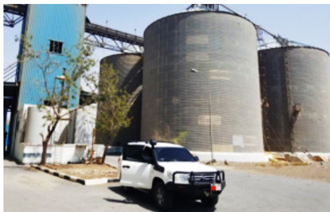
The Red Sea Mills in Al Hudaydah. Photo: WFP
