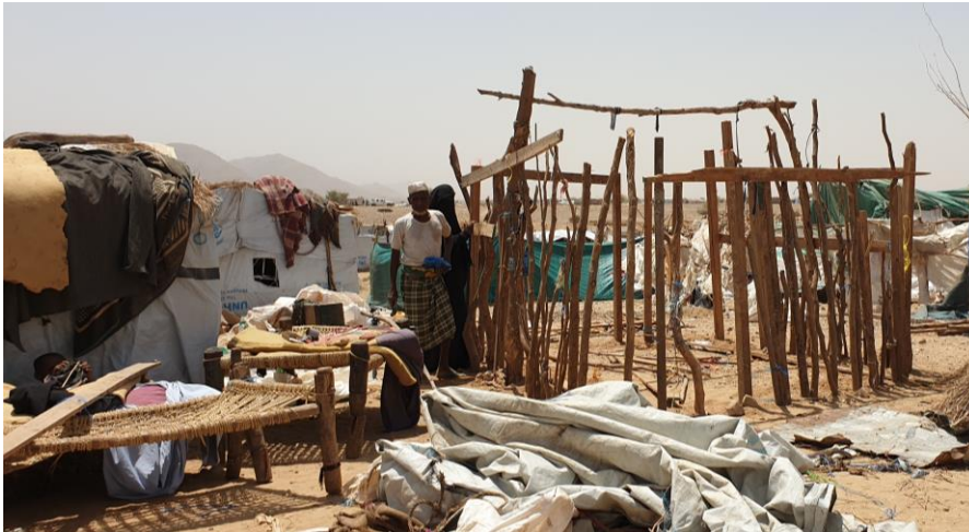
An elderly man with his wife trying to rebuild their transitional shelter in another site after they were forced to leave from a site they have used to be living for years as conflict advanced closer to their location in Abs district of Hajjah Governorate. © Shelter/NFI/CCCM Cluster/Monir AISobari.
